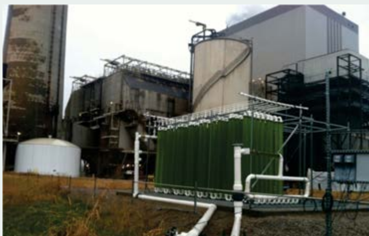
CERC researchers are exploring reactor designs for algae growth in a demonstration facility installed at Duke Energy's East Bend power plant at Rabbit Hash, Kentucky, United States.
