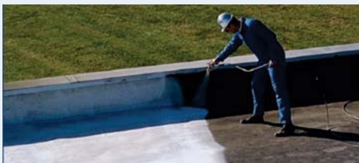
Research on white (cool) roof coatings is increasing cool roof performance, which facilitates greater market penetration that could result in significant energy savings.
