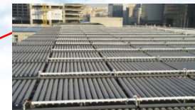
Solar water heating system
