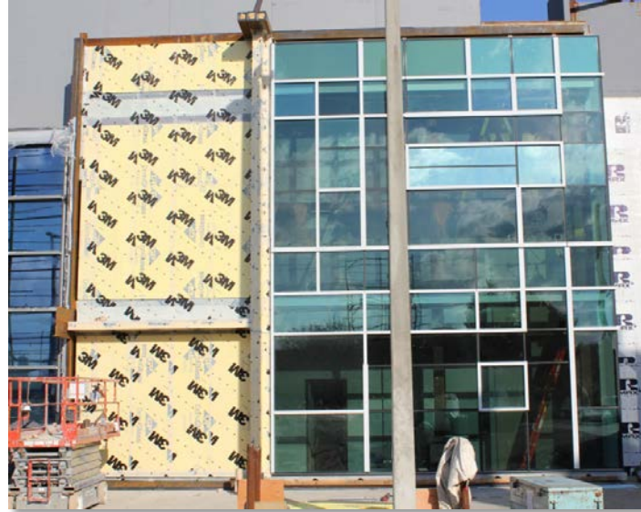
Substrates: exterior grade drywall and steel
