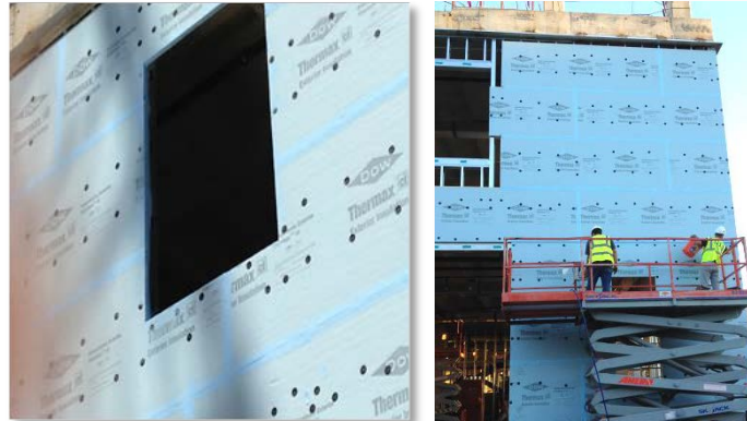
Substrates: foil-faced polyisocyanurate board insulation and steel
