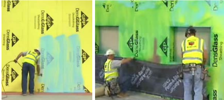
Typical asphalt-based self-adhered membrane Primer required over substrate
