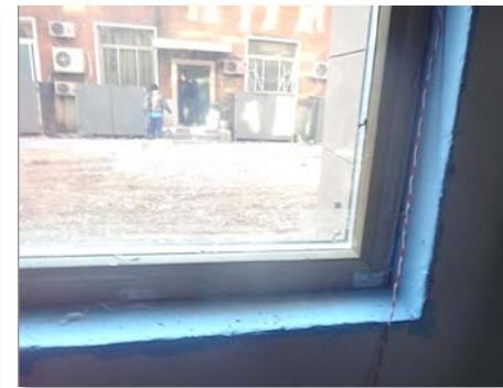
Installed liquid flashing
