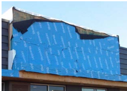
Failure can occur if primer is not adequately dried
