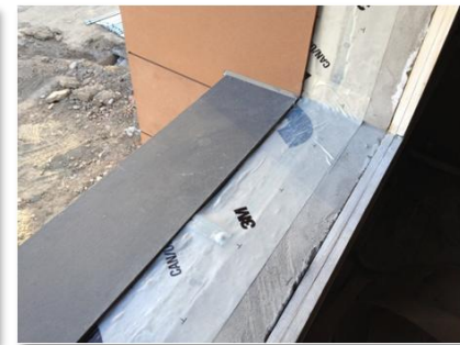
Membrane as flashing
