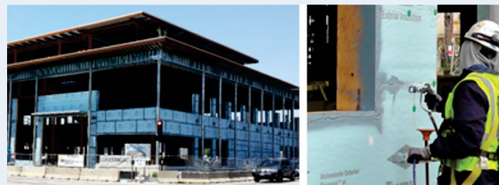
Demonstration building (left) with liquid flashing (right) sealing the gaps around penetrations and joints
