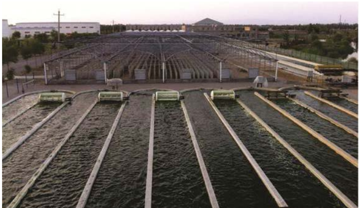
Demonstration of open pond microalgae cultivation at ENN research facility in Langfang, China, using CO 2 from a coal gasification plant
