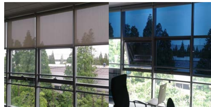
The performance of low-emittance windows with manually operated roller shades (left) being compared to automated switchable electrochromic windows (right) in the Saint-Gobain Research Shanghai building
