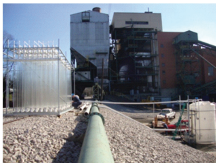
Photobioreactor under construction at Dale Power Station in Kentucky
