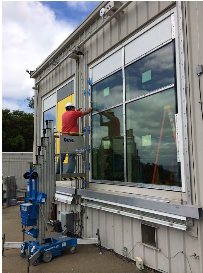
Figure 5: Installation of Sage electrochromic windows (righthand windows in the photo) in the LBNL Advanced Windows Testbed.
