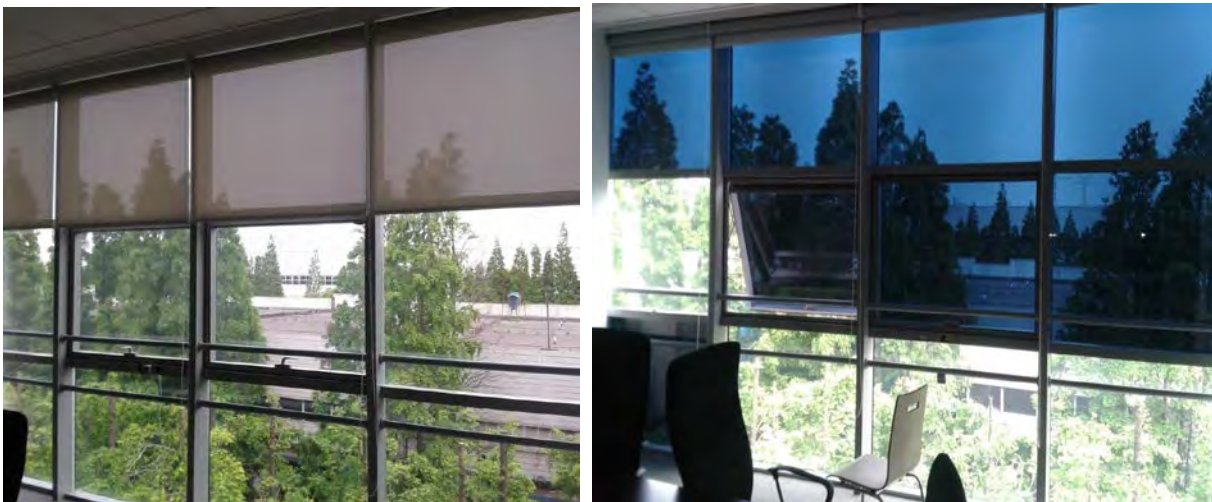
Figure 6: The performance of low-emittance windows with manually operated roller shades (left) are being compared to automated switchable electrochromic windows (right) in the Saint-Gobain Research Shanghai building. Each of the three rows of electrochromic windows are switched independently according to daylight availability and the position of the sun. The windows can be opened manually for ventilation.
